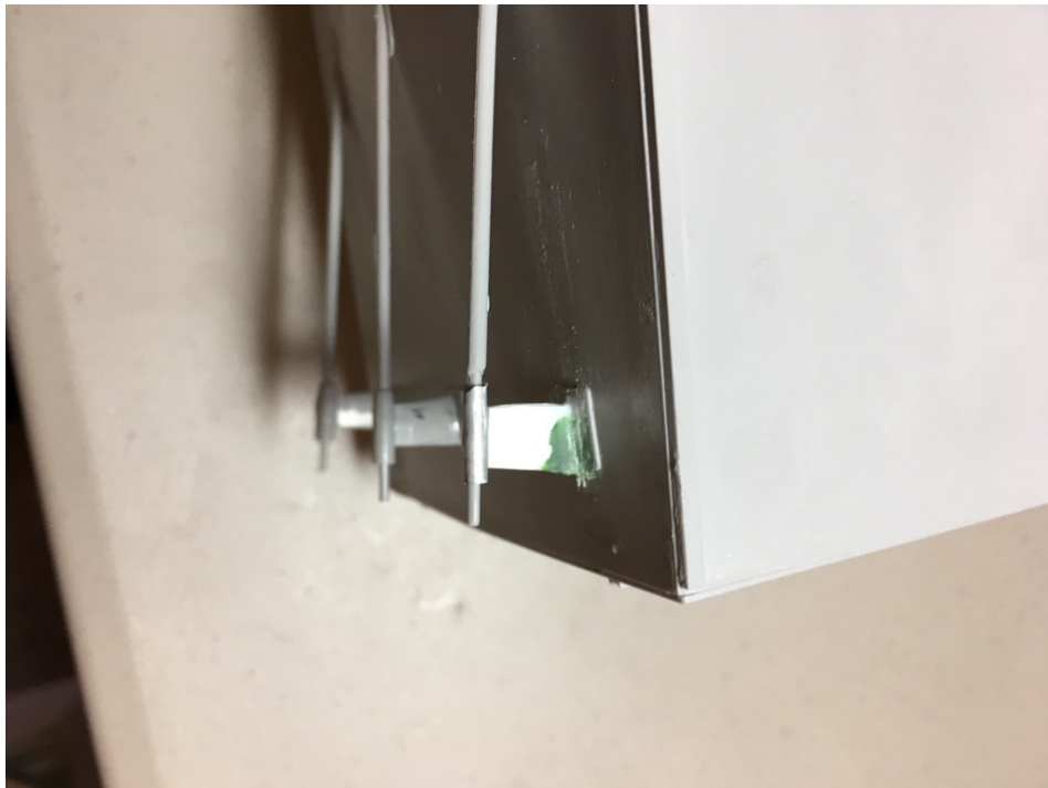
Figure 3. The replacement strut before sanding and primer.
